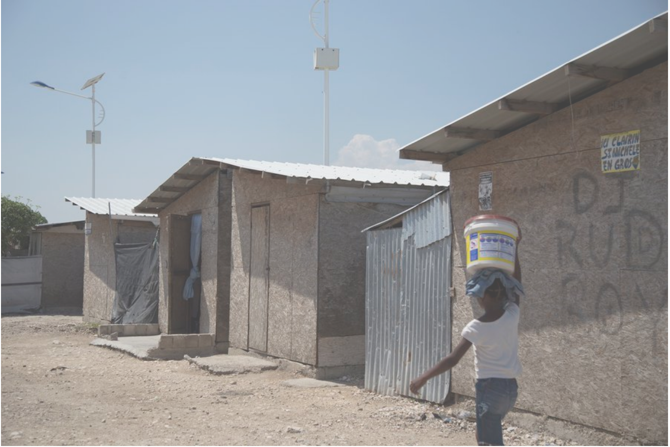
Transitional shelters like these on the outskirts of Port-Au-Prince, paid for by the Red Cross, typically last three to five years. (Marie Arago, special to ProPublica)
